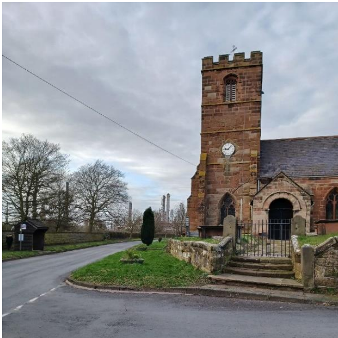
Image 4 – Church of St Mary, in Thornton-le-Moors Conservation Area (Grade I Listed Building)
